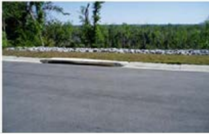
New Drain Inlet
