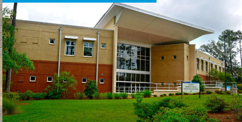
Building Building 960, Room 200A
