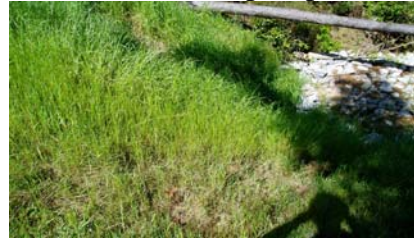
Outlet with Rip Rap
