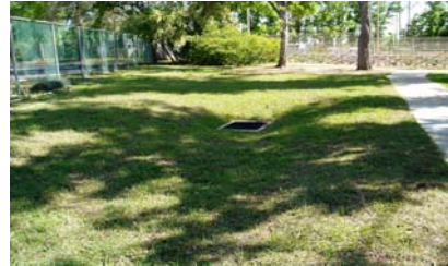
New Drain Inlet
