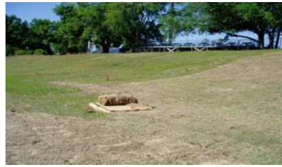
Drainage pipe area with new inlet
